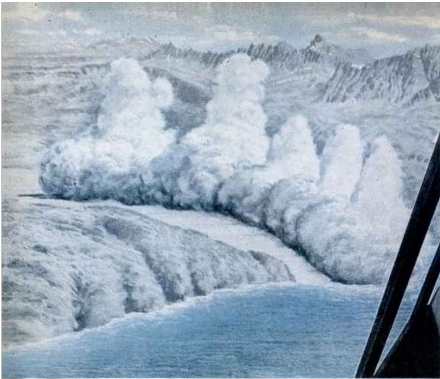
In a matter of milliseconds, five nuclear bombs will blast open a new harbor in Alaska. The channel will be 1800 feet long and 750 feet wide; the inner harbor, about a half mile long and a quarter mile wide
